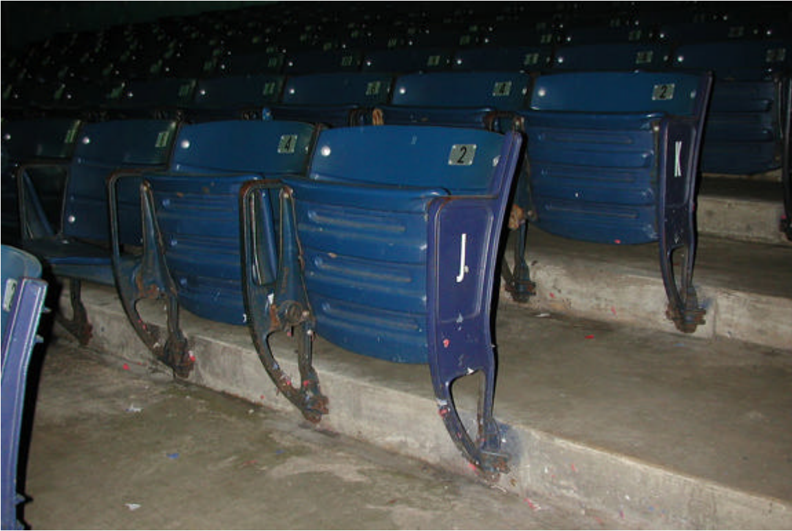
Original riser-mounted cast iron seating
