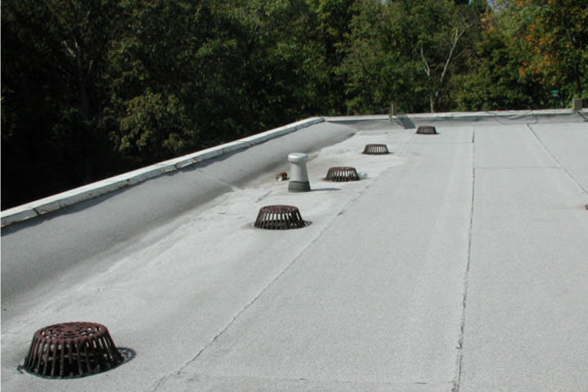
Roof Drains over Stage House. Main roof is in good condition.
