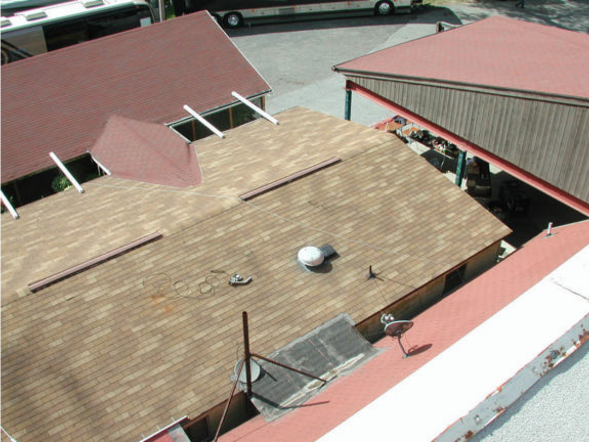
Dressing Rooms in manufactured building behind stage. Catering decks, bus parking beyond
