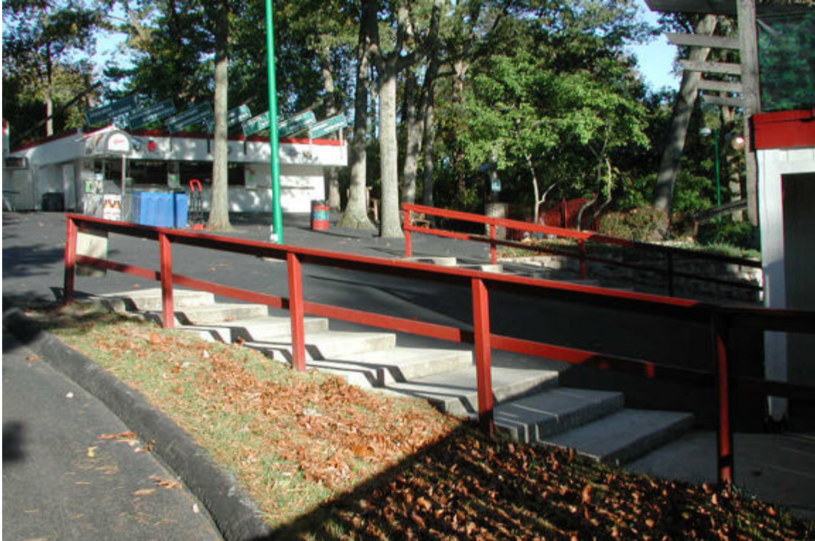
Steps down to restrooms at Main Entrance Plaza. Note slopes.
