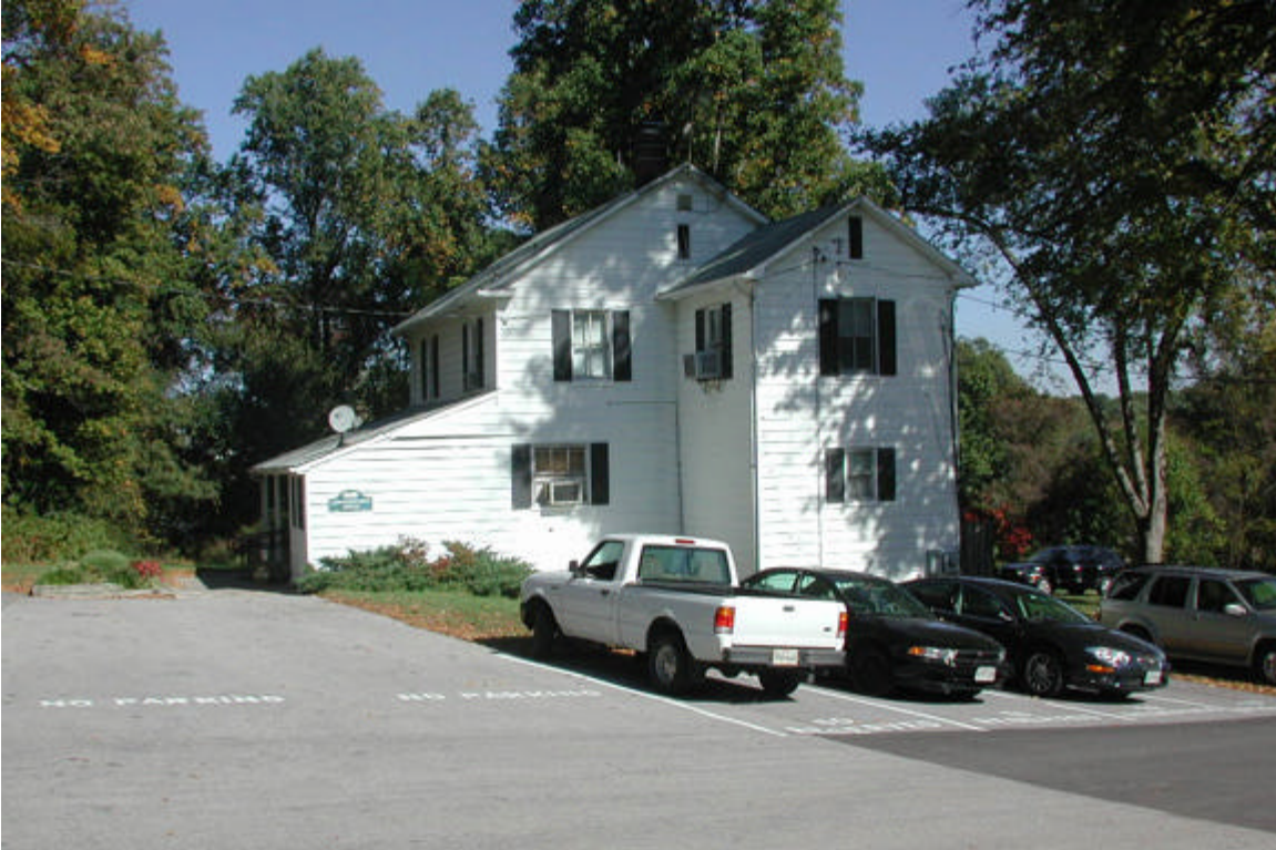
Administration Building and parking
