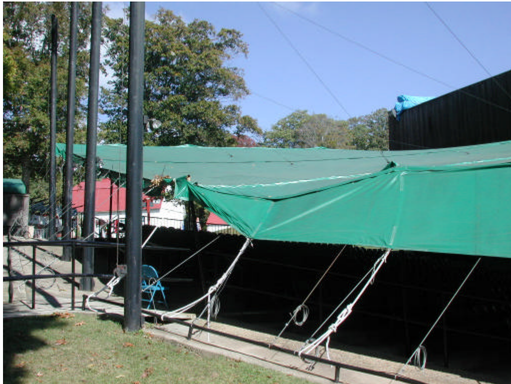
Guying for Loge tents at grade. Note bridge over stormwater swale.
